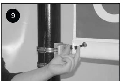
6) Secure the banner with nylon cable ties through eyelet on banner and through small hole in arm casting. Do not over-tighten as this may cause banner to wrinkle, snip excess cable off with snips. This holds banner onto brackets acting as a safety measure.
